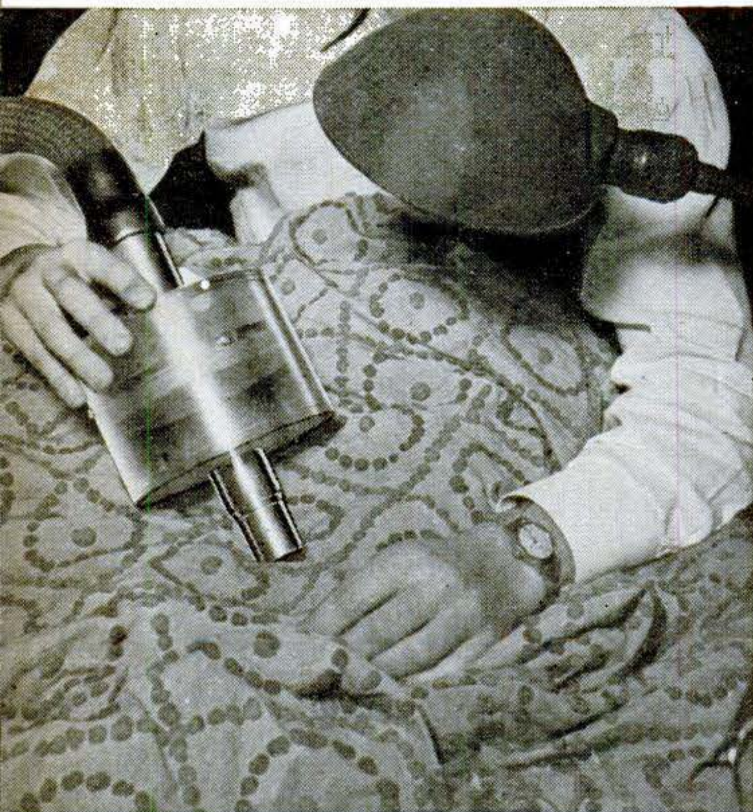
1. Searching for telltale hairs, Dr. Kirk goes over a bedspread with a special vacuum attachment. Hairs will be caught on a porous disk through which air but not dirt can pass.
